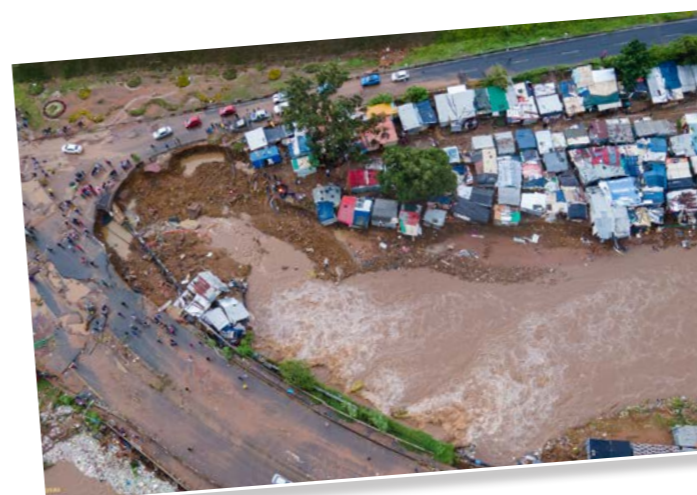
A drone image taken on 12 April 2024 of the hole created by the river changing course and of the containers washed across the road (Source: Yajur Chotai)
